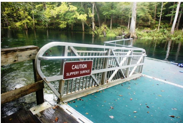
Figure 2. Caution Signage 'Slippery Surface'
