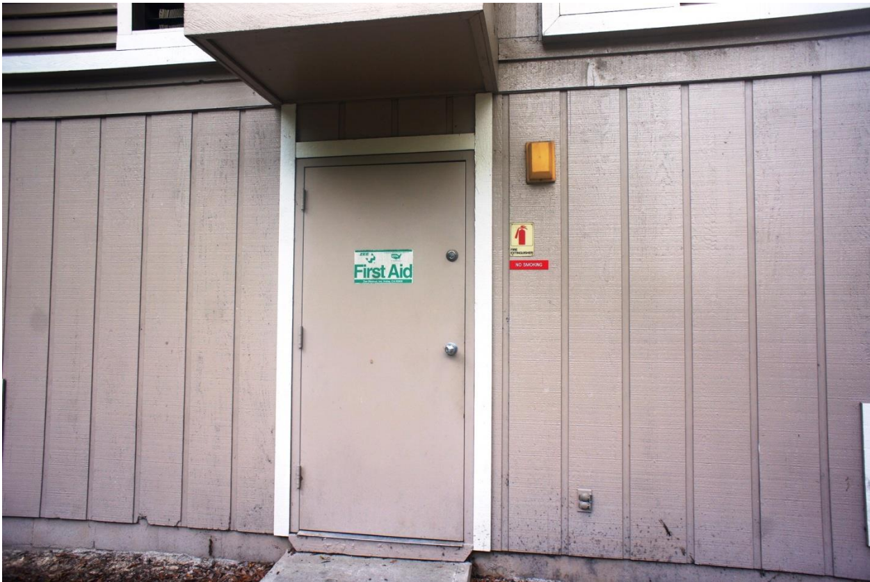
Figure 8. Emergency room closed
